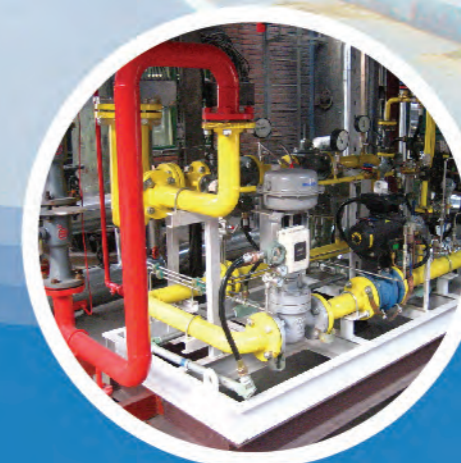
燃料供应系统撬块 Fuel Train System in Skid
