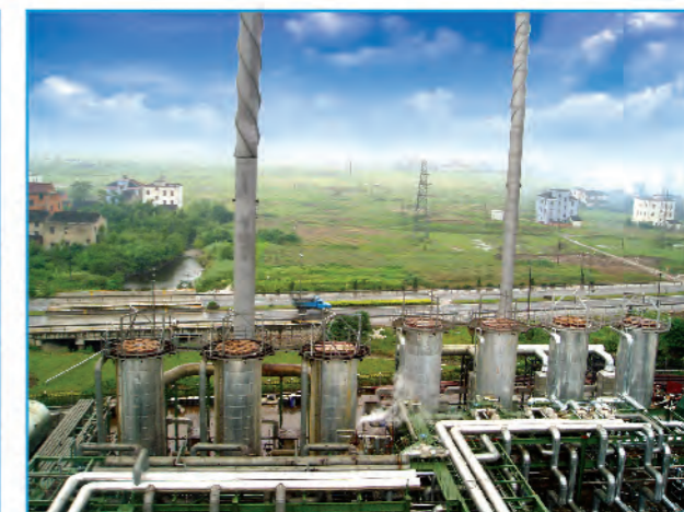
浙江桐昆集团聚酯工程7X1000万大卡热媒站 7 sets of 10 Mkcal/h hot oil heater station for polyester plant, Zhejiang Tongkun Group.
