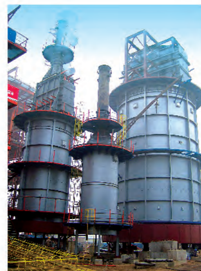
华北石油管理局苯乙烯项目循环苯加热炉 Benzene-cycling heater for benzene styrene project of North China Petroleum Administration Bureau
